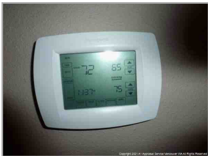
Utilities On (Thermostat)
