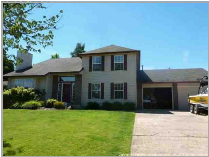
Front; Hardi Plank Siding, vinyl windows and composite roof
