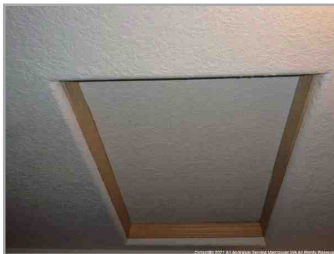
Attic/Scuttle Access (Primary Bedroom Closet ceiling)
